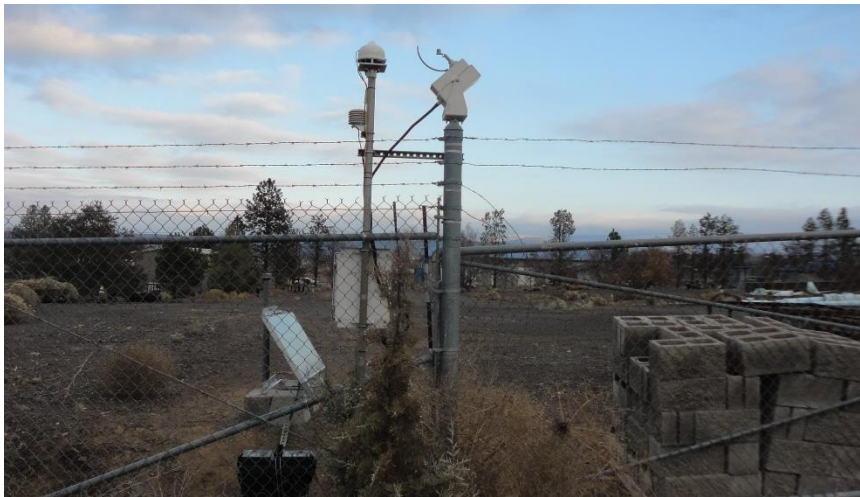
Figure 7. View of the station facing East.
