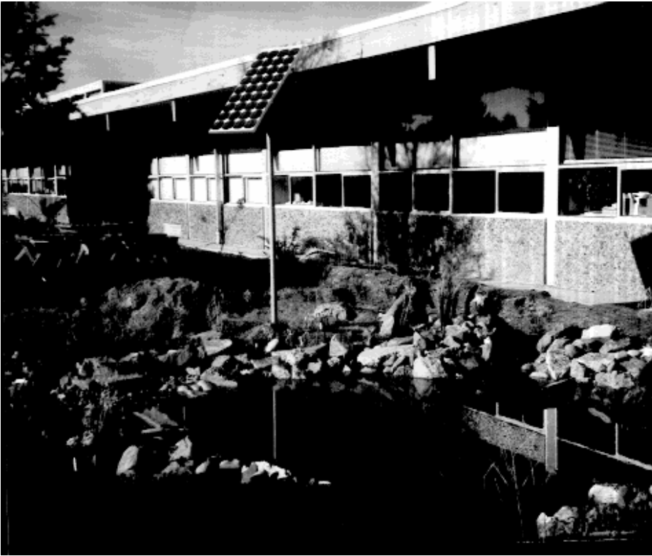
Photovoltaic Array powers nature-scaped wildlife habitat at Rowe Middle School in Milwaukie, Oregon
