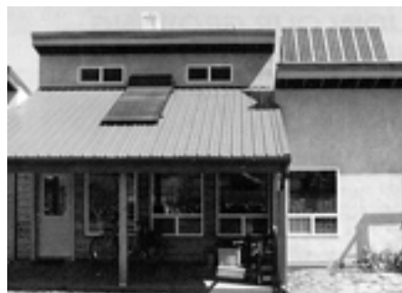
PV and solar thermal. Picture from the Energy Service Company web site: www.efn.org/~esco .
